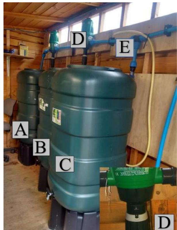
**Figure 5:** Irrigation system consisting of A) calcium feed tank B) starter feed tank C) fruiting feed tank D) dosatrons (1:64 injection) and E) pre-acidified water supply (pH 5.5)
